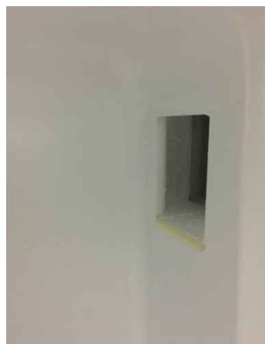
Air supply outlet of refrigeration room
